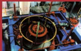
Test Facility - Lid Lift
