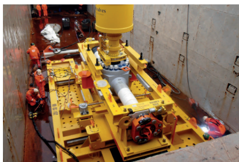
Subsea Riser Positioning
