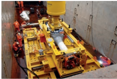
Subsea Riser Positioning
